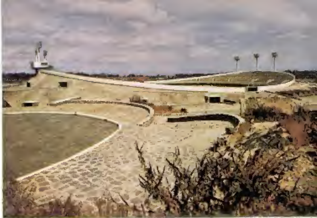
Huge Olympic Stadium was designed to resemble the crater of a volcano. High sides are opposite the mid-field marker, giving more of the spectators seats on the 50-yard line. Seating capacity of the stadium is 103,000
